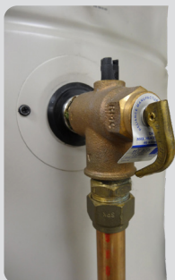
TPR position - top of cylinder
