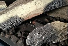
Ensure that there are NO granules placed directly over the Burner Ports to the front and back of the Pilot Burner to the Flame Rods.
