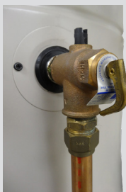
TPR position - top of cylinder
