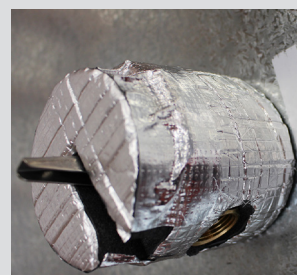
Insulated TPR valve for the 250 and 300 L cylinders
