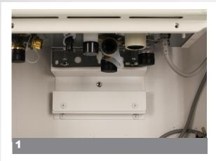
Take the EF26 lower adapter from the kit and fit over the existing installed bracket as shown above.
