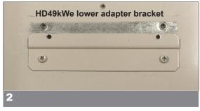
From the kit, attach the HD49kWe lower adapter in place. Note position and orientation as pictured.
