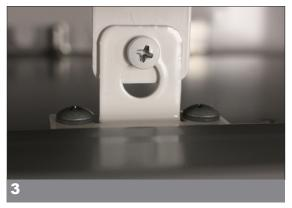
Fit the HD49kWe top mounting bracket to unit, lift unit into box, secure back section into metal pocket, and screw top section in place.
