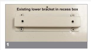
Remove the existing lower bracket inside the recess box and discard (recycle).
