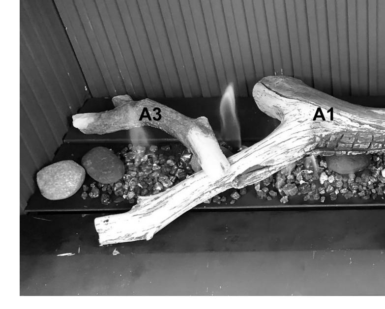
We recommend identifying the log sections before installation—lay them on the floor in a configuration resembling the above. This will ensure you're not forcing incorrect log pieces onto the burner supports and scratching the paint.
