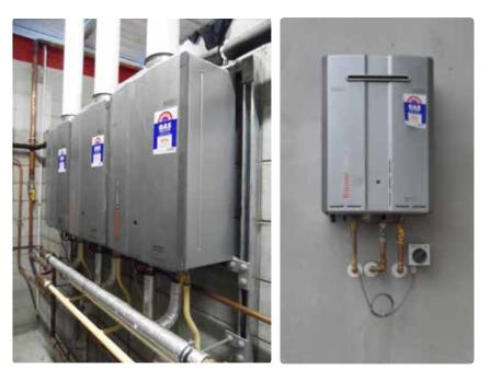
EFi250 condensing manifolded units operate more efficiently than standard HDi200 units, saving on operational and life cycle costs.
