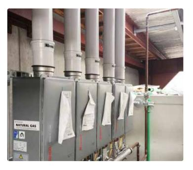
Rinnai INFINITY HDi200 units can be installed almost anywhere. These units were installed in a roof space and flued through the roof.
